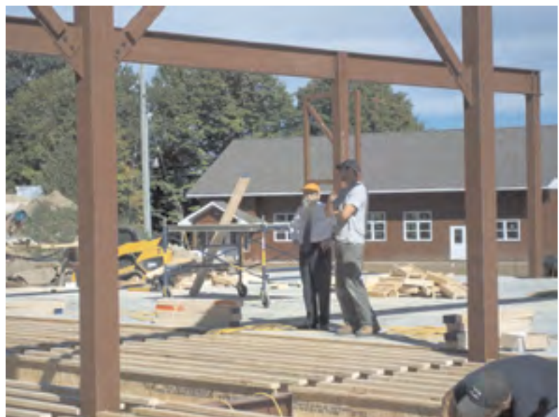
Construction of the kitchen / dining room. Shul / Auditorium can be seen in the background.
